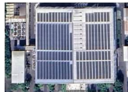
Solar Power System of Production Base 1
