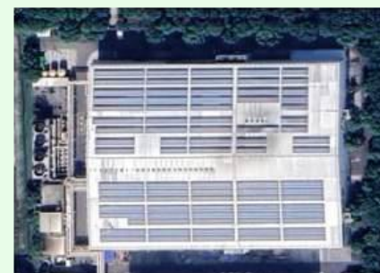
Solar Power System of Production Base 2
